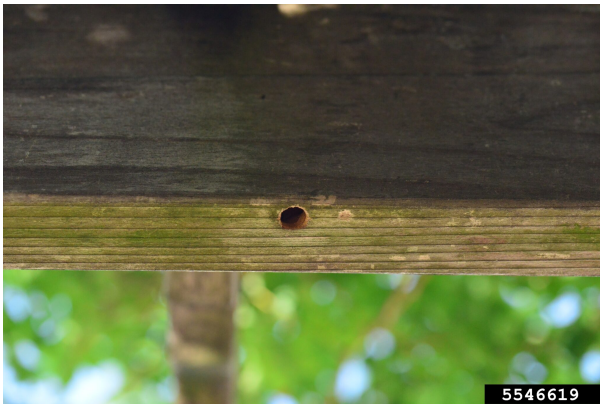
IMAGE 1: Carpenter bee entrance holes are distinctive because they are perfectly round and about the size of your pinky finger. Photo by David L. Clement, University of Maryland.
